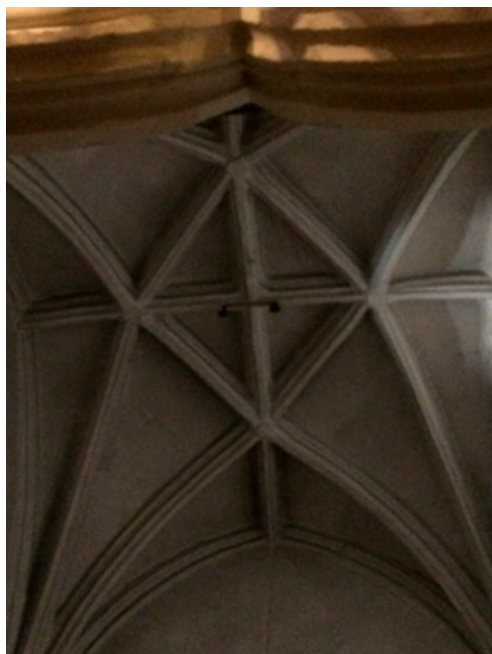
Fig. 10. Vault of the "Ribadeneira" chapel, church of San Justo y Pastor, Toledo. Chapel completed in the late fifteenth/early sixteenth century. Source: Costanza Beltrami
